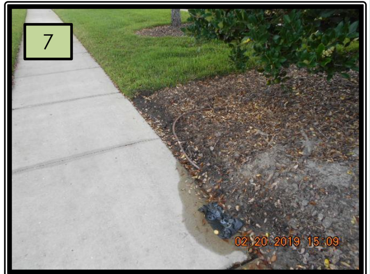
7. Reference Pic (7) Broken irrigation was found in the landscape beds at the amenities center.
