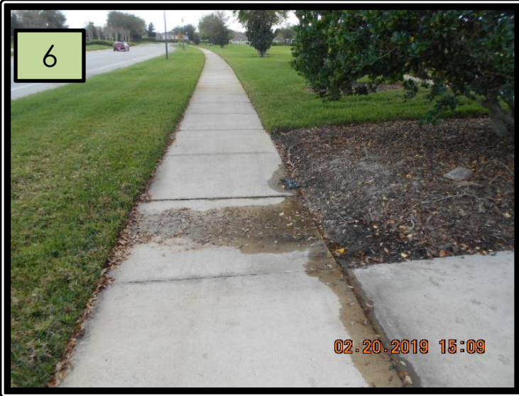
6. Reference Pic (6) Located at the amenities center there is a irrigation repair that needs to be addressed as the water is leaking onto sidewalk.
